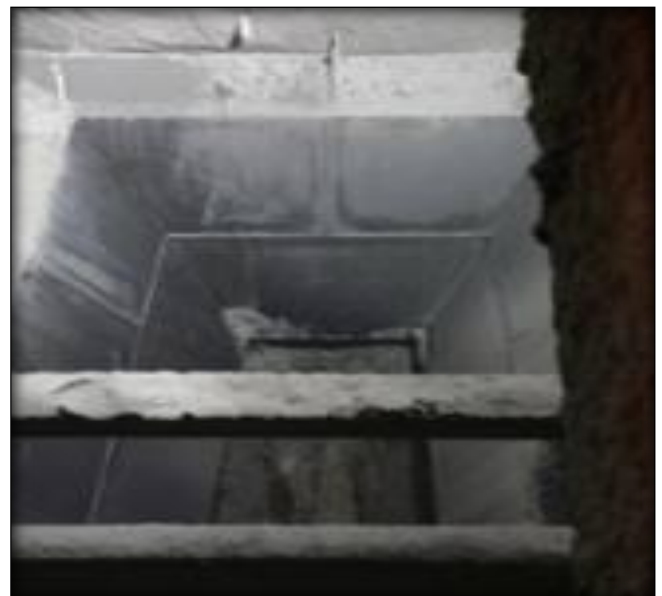
Clear chute with Self-Cleaning liner
